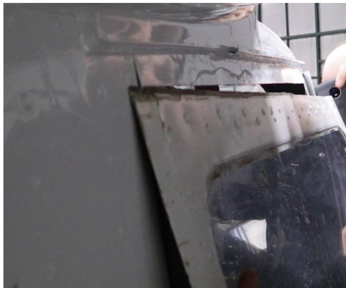
Figure 8: Emergency window topside installation
