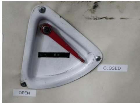
Figure 16: Safety action; marking of the handle position
