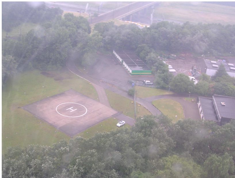
Figure 5: Overview of heliport
