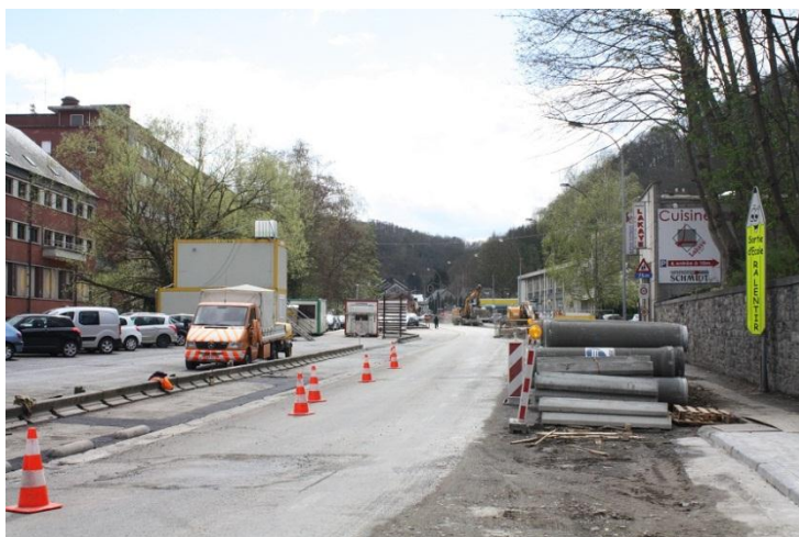
Figure 1: view of the works rue du Houyoux
