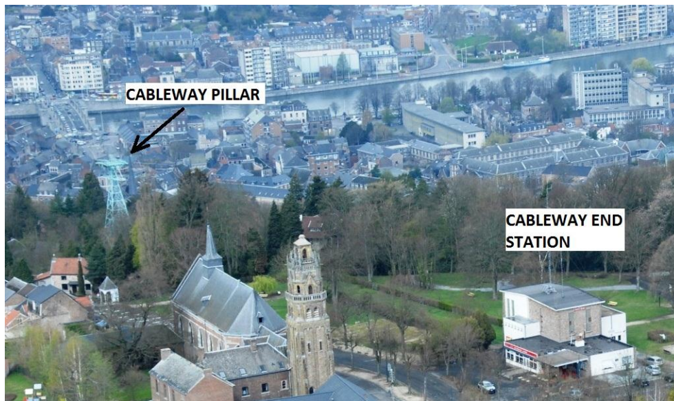
Figure 26: Example where cables are invisible due to a dark background.
