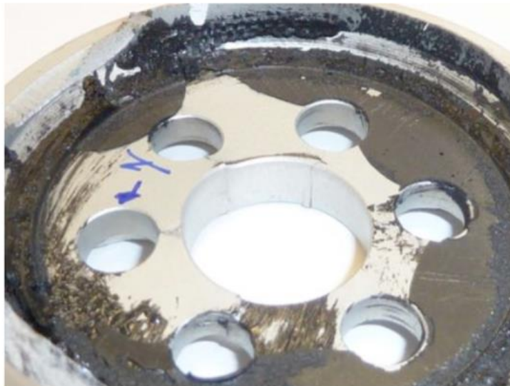
Figure 10: view on the fixation ring and the cracks in the weakest section near each hole;
